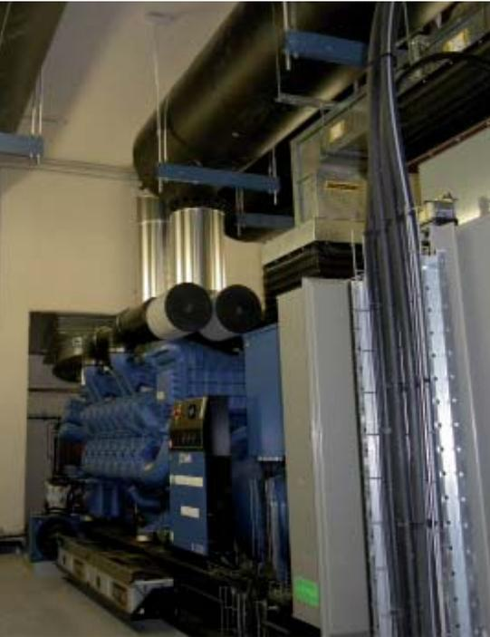
In France, the hospital in Saumur can accommodate 455 patients. The site has a back-up power plant comprising two 2,200 kVA SDMO® generators.
