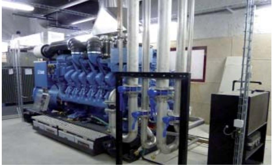
The University Hospital has six 2,000 kVA generators used as back-up for mains power, and during Peak Day Withdrawal. The installation of this power plant (carried out to replace the former, obsolete plant) was conducted in strict adherence to the work schedule and the sound level constraints relevant to the site: the date of installation of each component and the timescales allocated for carrying out trials were scrupulously respected, so as to avoid any cuts in power or back-up
